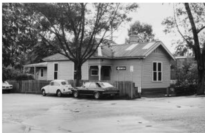
Station Master's House, Eltham Railway Station, August 1983 Photograph - George Coop
