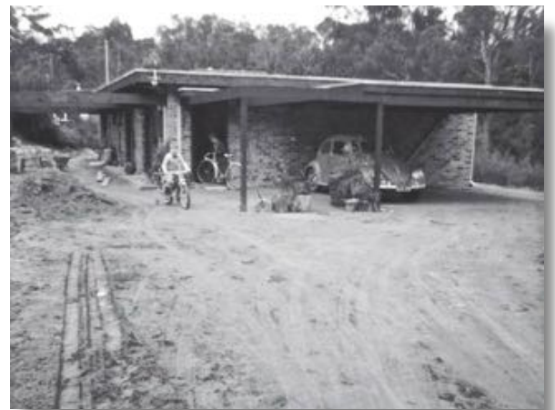
Work progressing on our house Photograph - Sue Bennett
