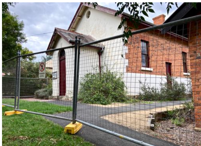
Former Eltham Court House - all fenced off Photograph - Jim Connor
