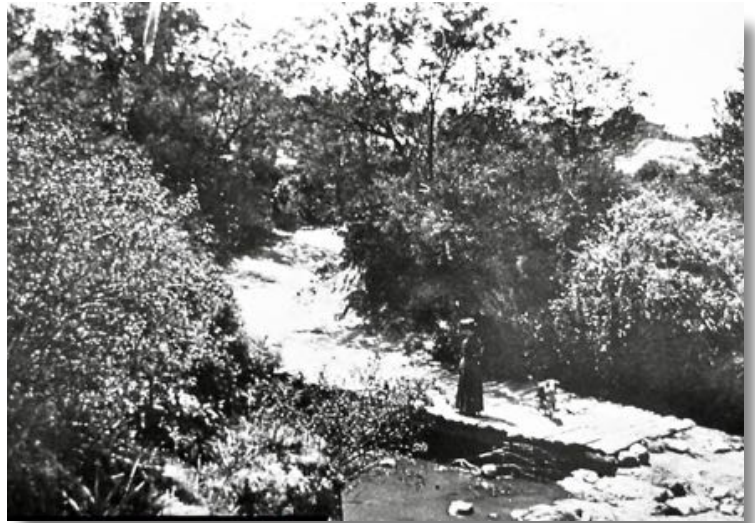
Kaylocks Bridge c1895 Photograph - EDHS collection
