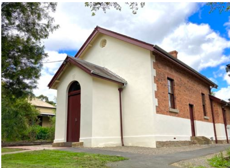
Eltham Courthouse - October 2021
