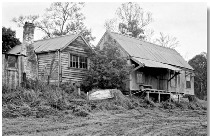
Falkiner Cottage, 1979, then situated at 19 Ely St., Eltham Photograph - Alan Baker - EDHS collection
