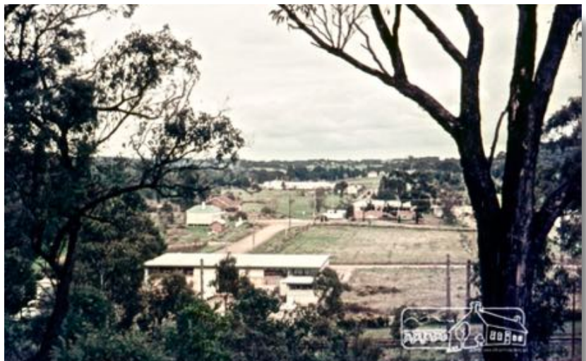
Looking south from Swan Street, Eltham, c.1965 Sibbel Builders factory is in the foreground Photograph - Russell Yeoman
