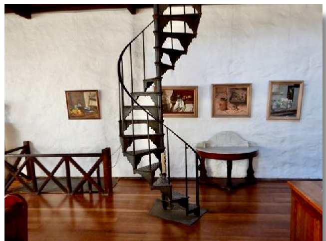
The cast-iron circular staircase
