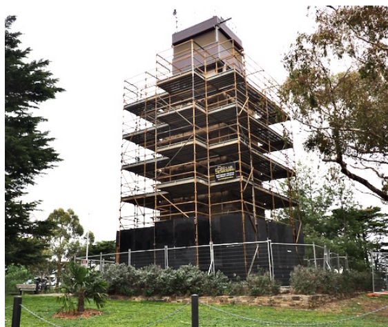
War Memorial Tower under restoration Photograph - Jim Connor
