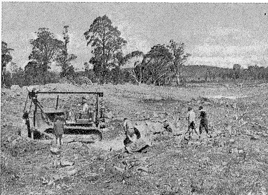
Start for Building of WADDAMANA CANAL
