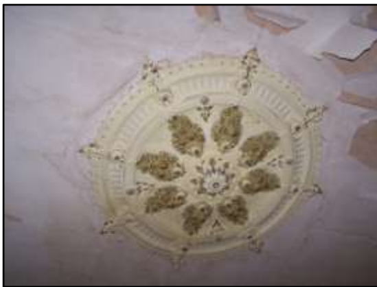
Source: David Fisher – Property Caretaker
