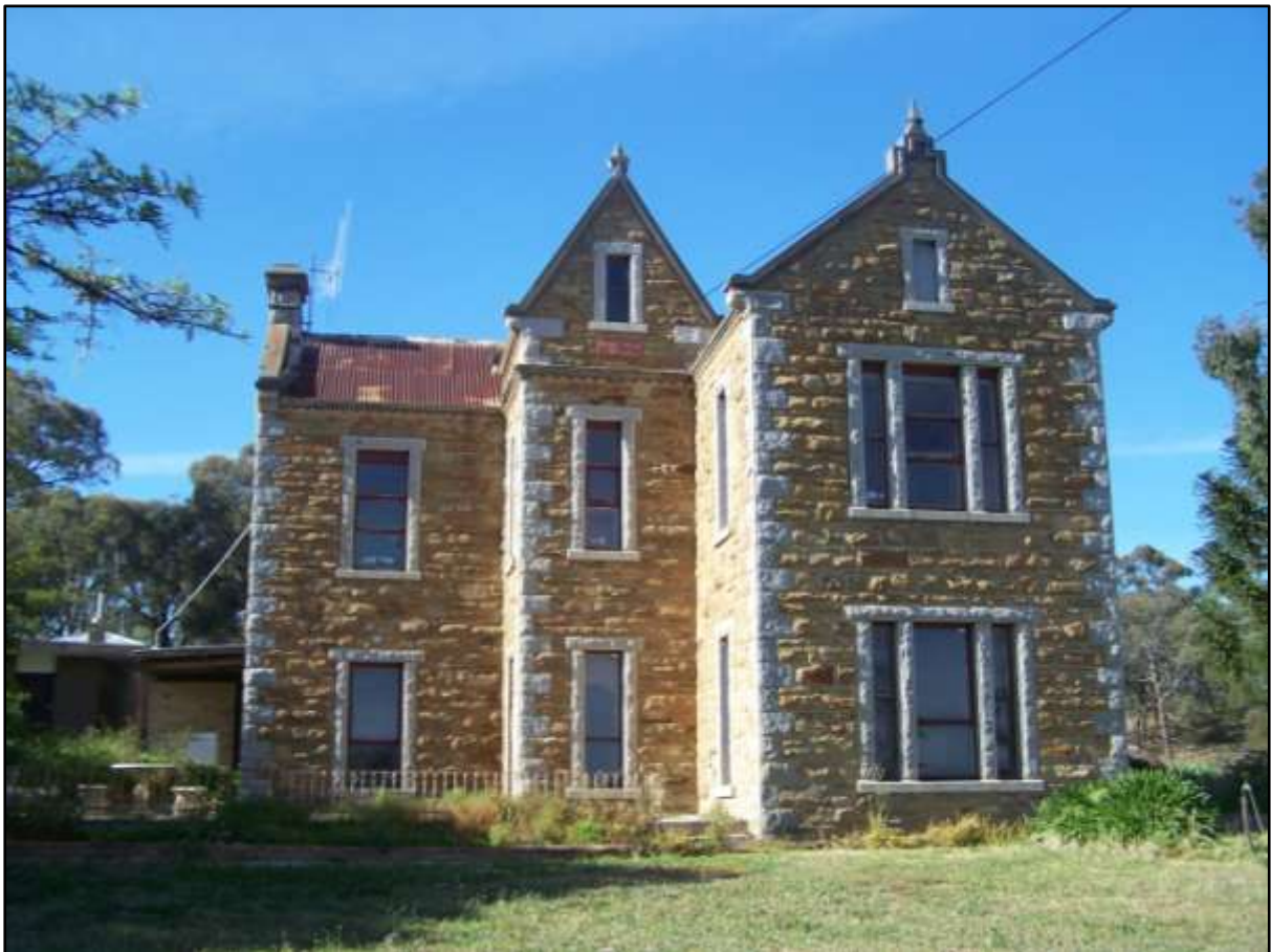
Source: David Fisher – Property Caretaker
