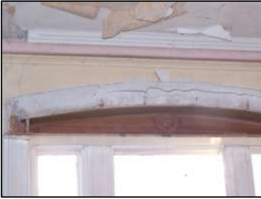
Source: David Fisher – Property Caretaker
