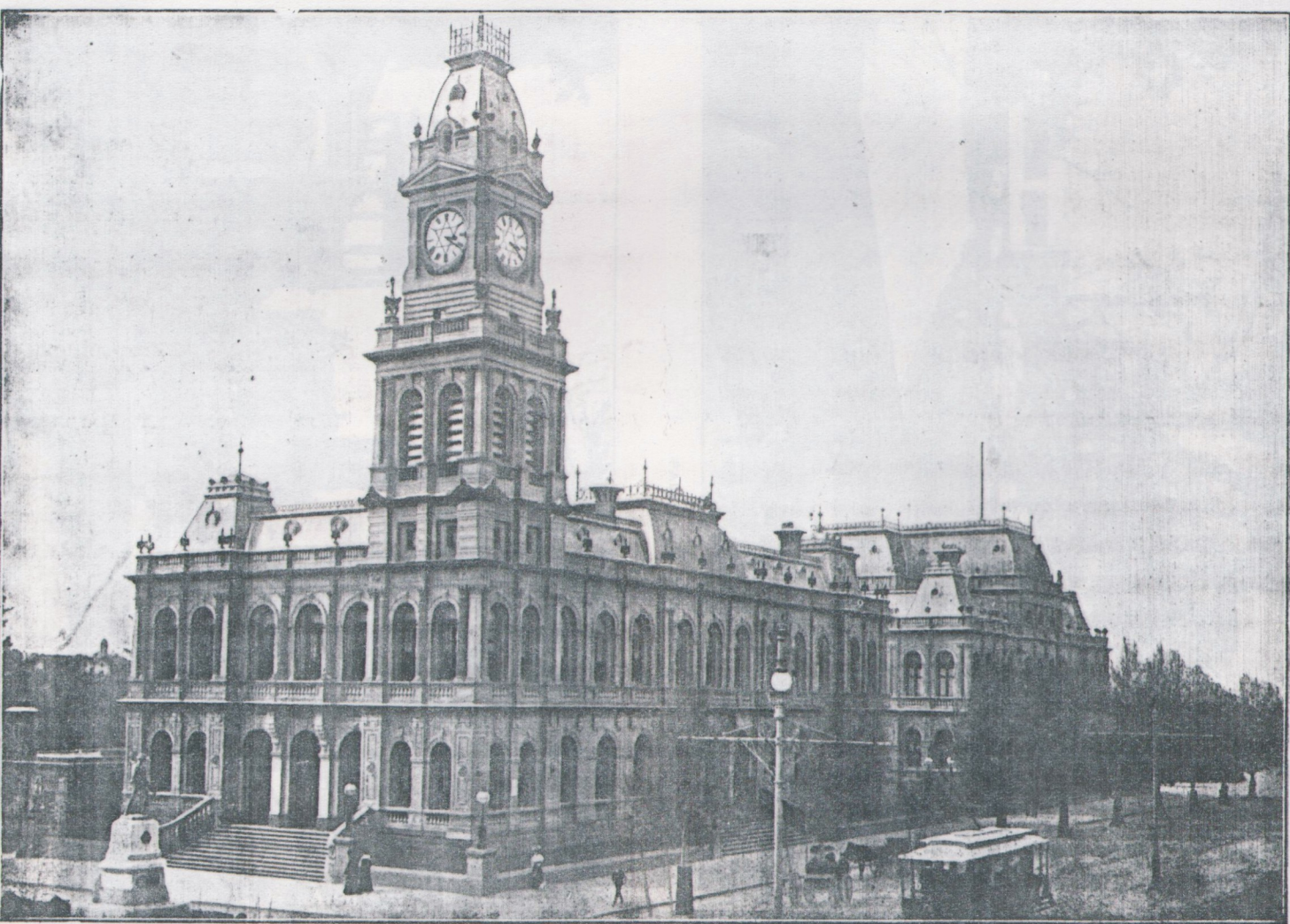
THE POST OFFICE and Law Courts
