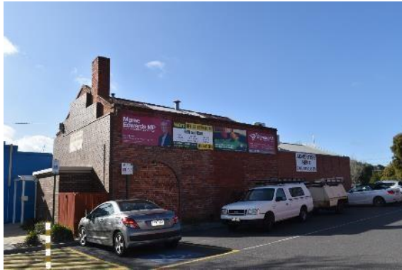
Figure 4. Golden Square Working Men's Club. Source: Minerva Heritage 2020
