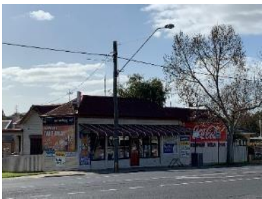
Figure 10. Former Howe's Fruit Shop on the corner of High and Maple streets
