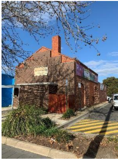
Figure 7. Working Men's Club, High Street
