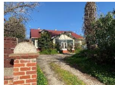
Figure 15. Interwar bungalow at 325 High Street
