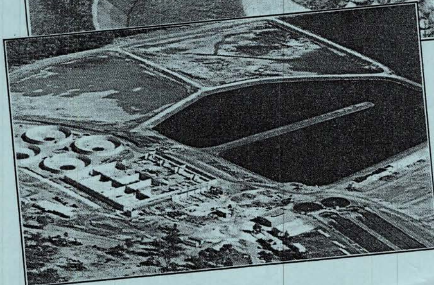
New Biological Nutrient Removal Plant at Bendigo
