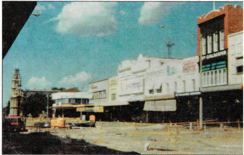
BUILDING: Construction of Hargreaves Mall began in February, 1982.
