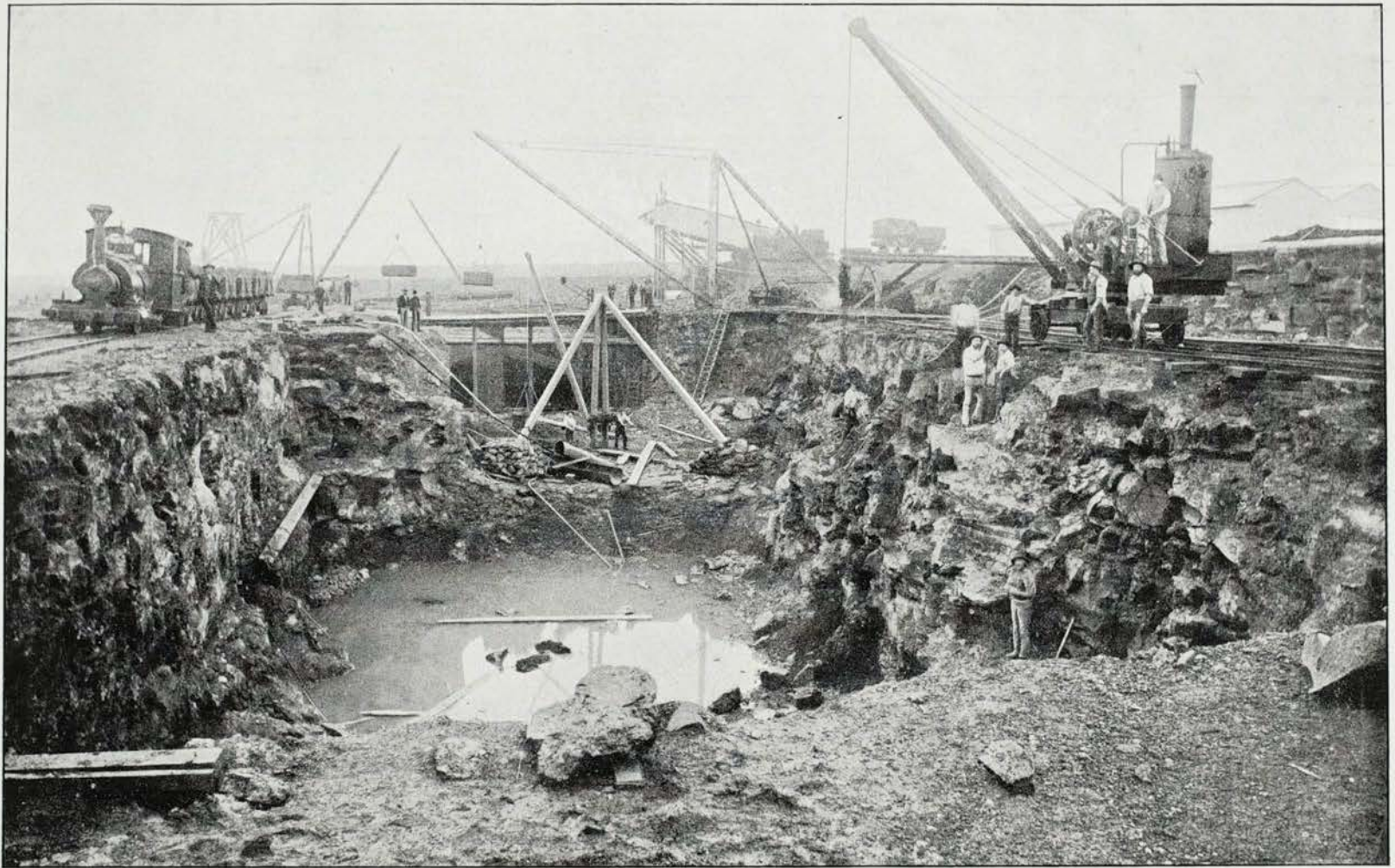
Excavation for Pumping Station, Spotswood
