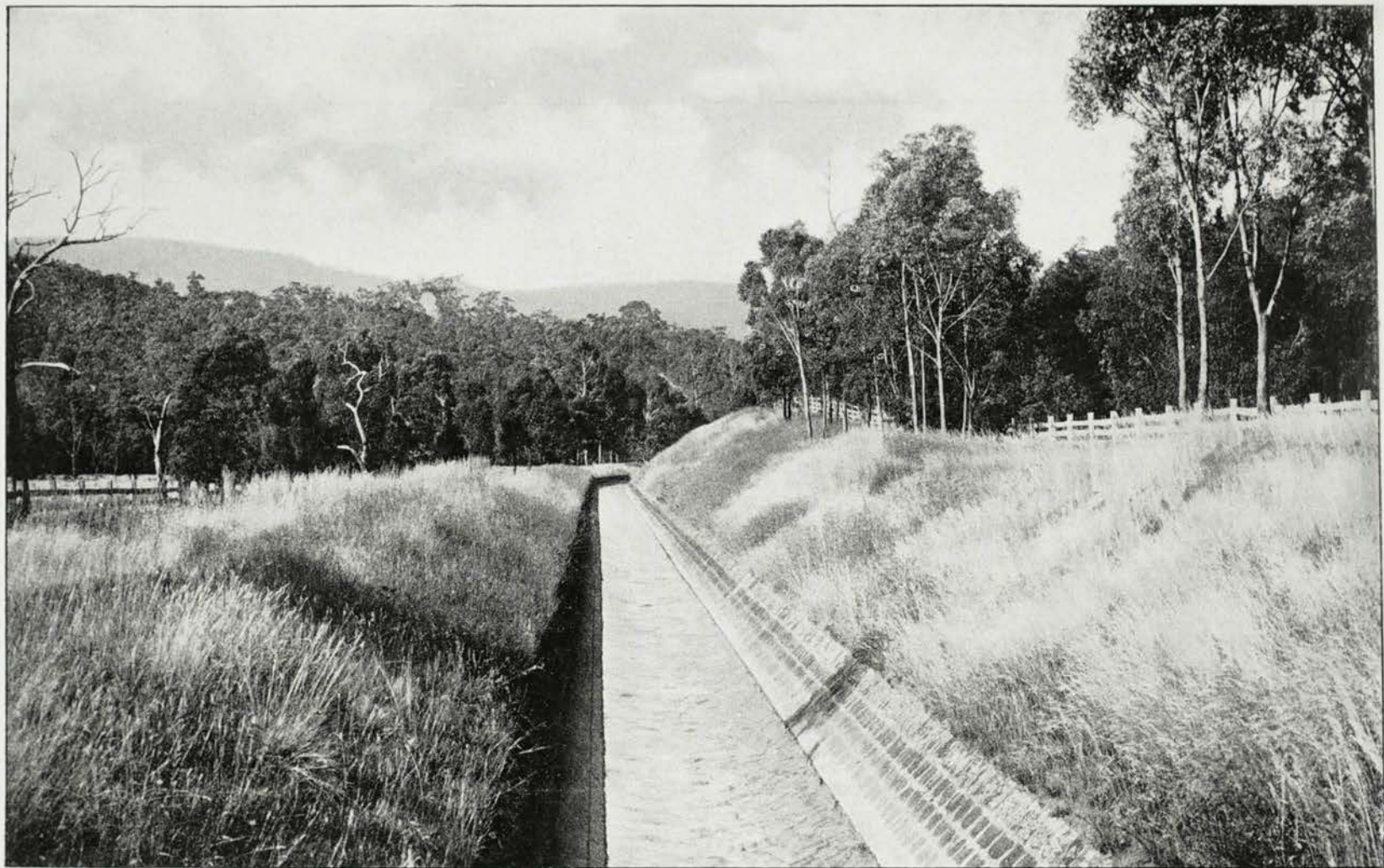
Clear Water Channel, Connecting Yan Yean and Toorourrong Reservoirs
