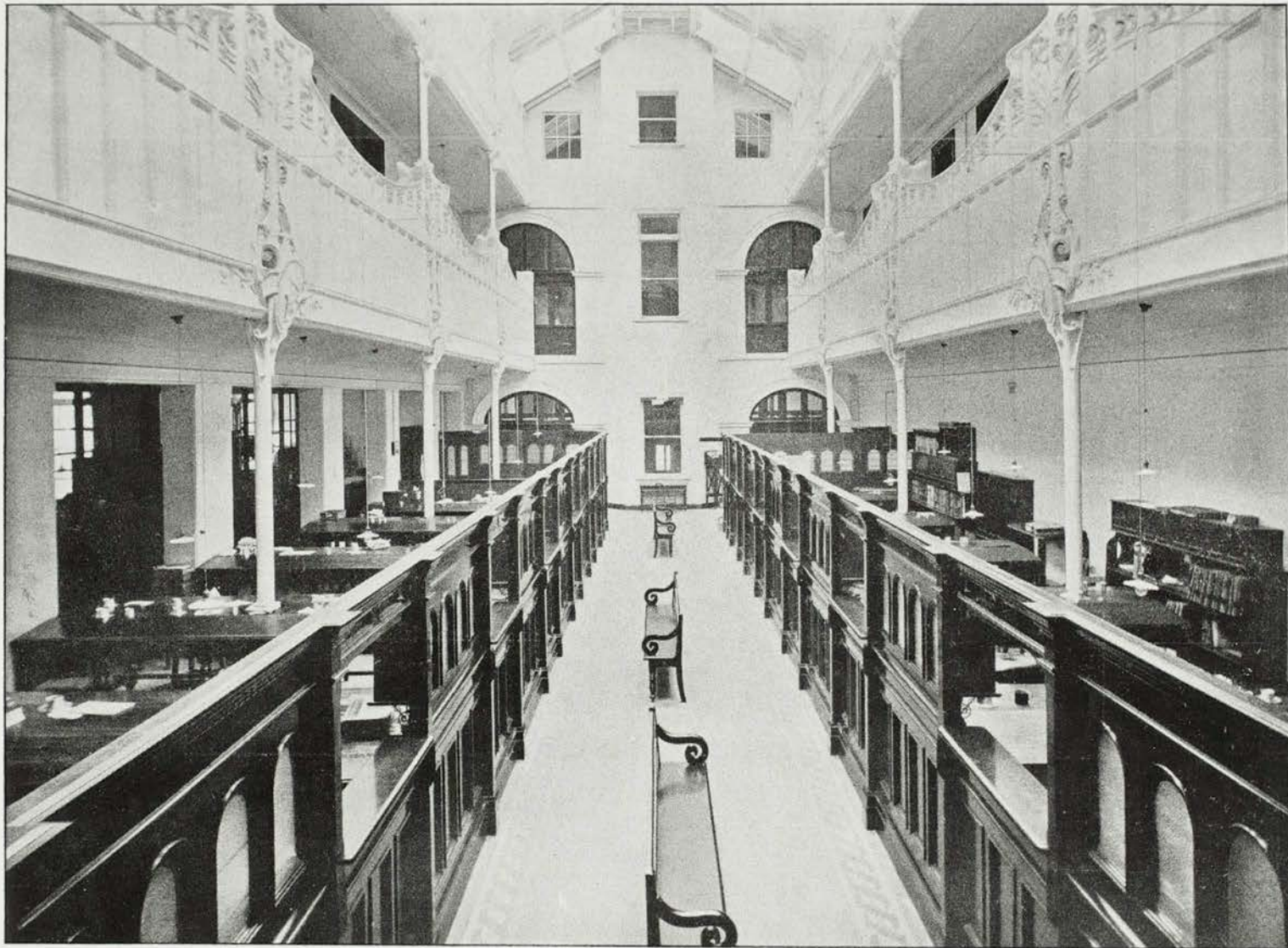
Interior of Rate and Accounts Office
