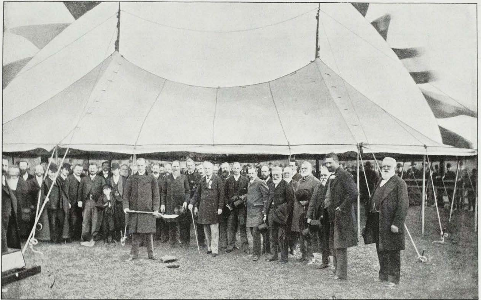
Turning First Sod of the Outfall Sewer
