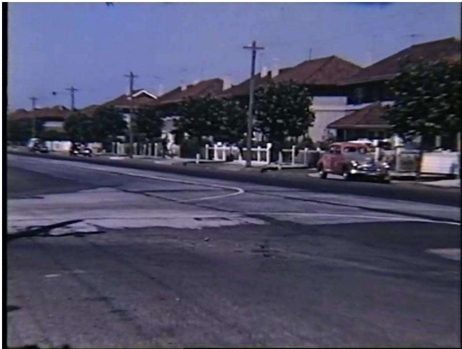
Aspect: View of the housing along the south side of Williamstown Road, looking east from the corner of Salmon Street.
