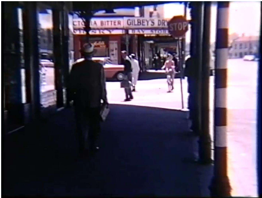
Aspect: Bay Street footpath looking north across Bridge Street to the Bay Stores Licensed Grocers. The Fountain Inn is in view at the top right of the photo.
