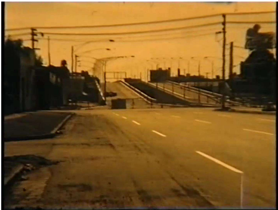
Aspect: View of the southern section of the King Street bridge, South Melbourne prior to its opening.
