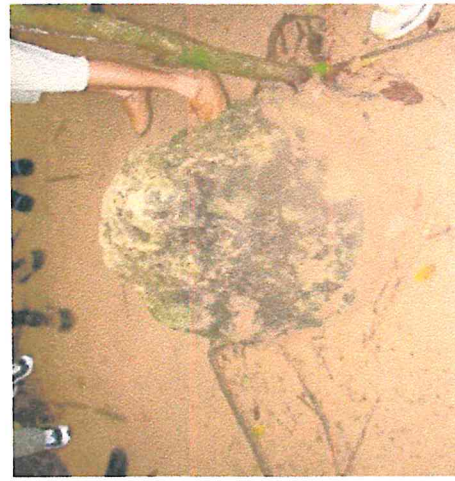
Air vent disguised as a termite mound.
