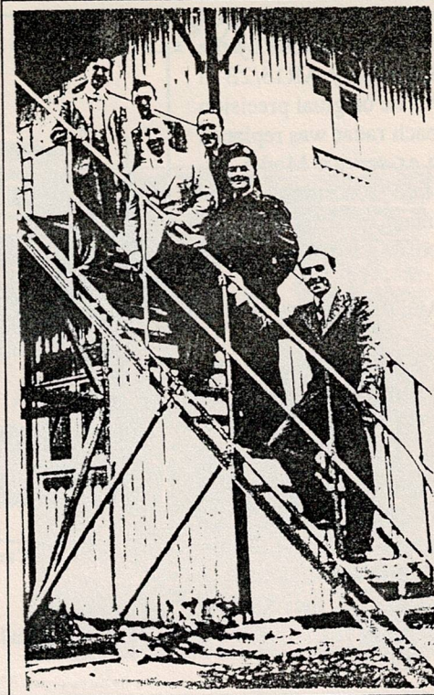
Aberporth-built tower with STC installation personnel. Author second up.
