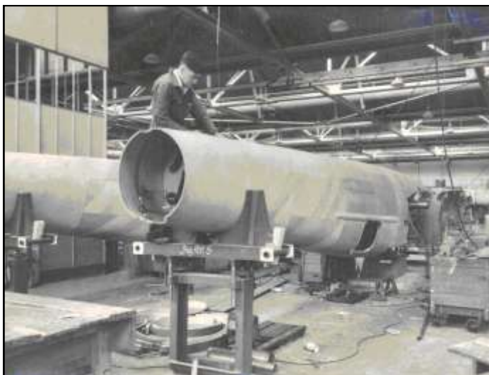
This photo shows the fuselage halves being joined together.
