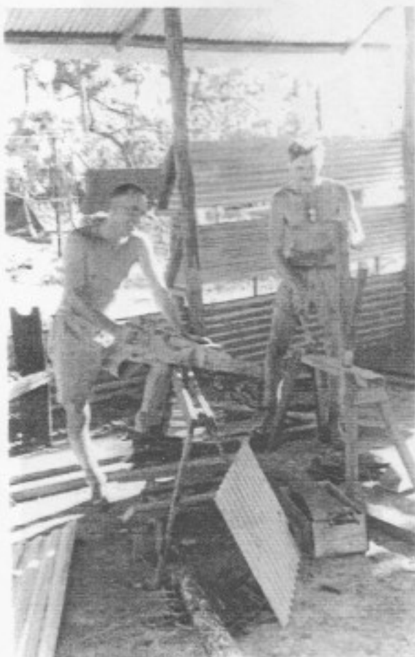
Carpenter Harold Peddy and mate at work on new chapel
