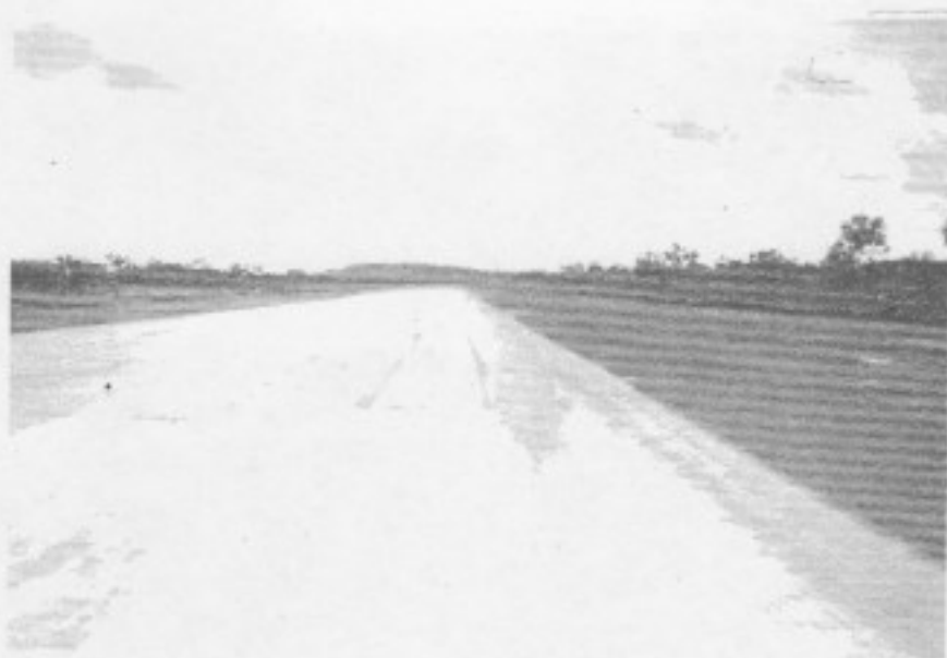
Coomalie Strip before final coat of dark gravel. 1943 (Photo Ian Ezzy)
