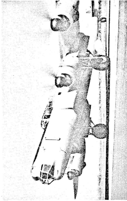
A Lincoln Mk.31 of No.10 Sqdn. RAAF. Note the 6ft 6ins extension to the fuselage forward of the cockpit. These aircraft were used for a variety of tasks but were mainly concerned with over water patrol duties. A total of 19 examples were built.
