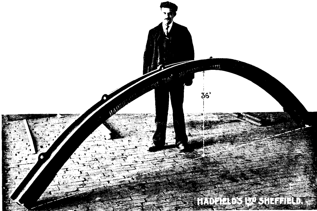
RAIL 15 FEET IN LENGTH. BENT COLD.
