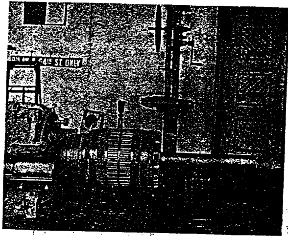
Fig. 10. The Other End of Shaft Than That Shown in Fig. 9 Supported by an Oak Pole With a Steel Tube Fitting Over the Shaft
