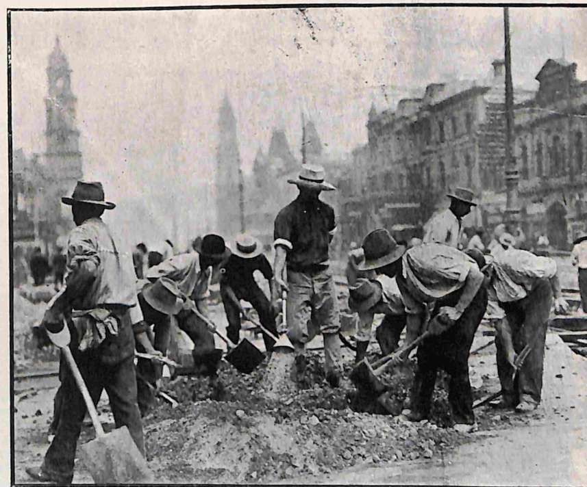
"CONCRETE-MIXERS" MAKING CONCRETE FOR THE TRACK BED IN KING WILLIAM STREET.
