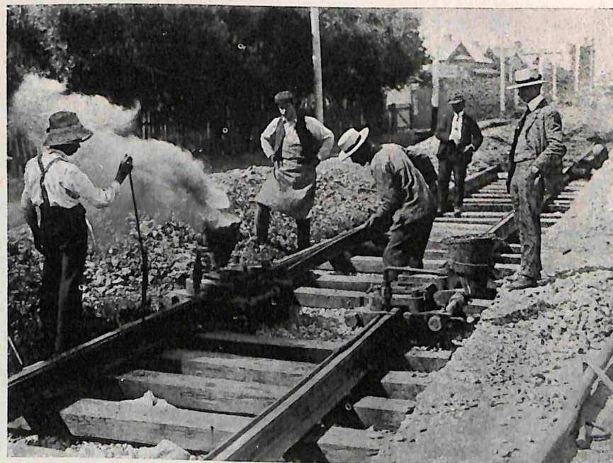
WELDING THE RAILS BY THE "THERMIT" PROCESS. THIS ENSURES A SMOOTH JOINT.
