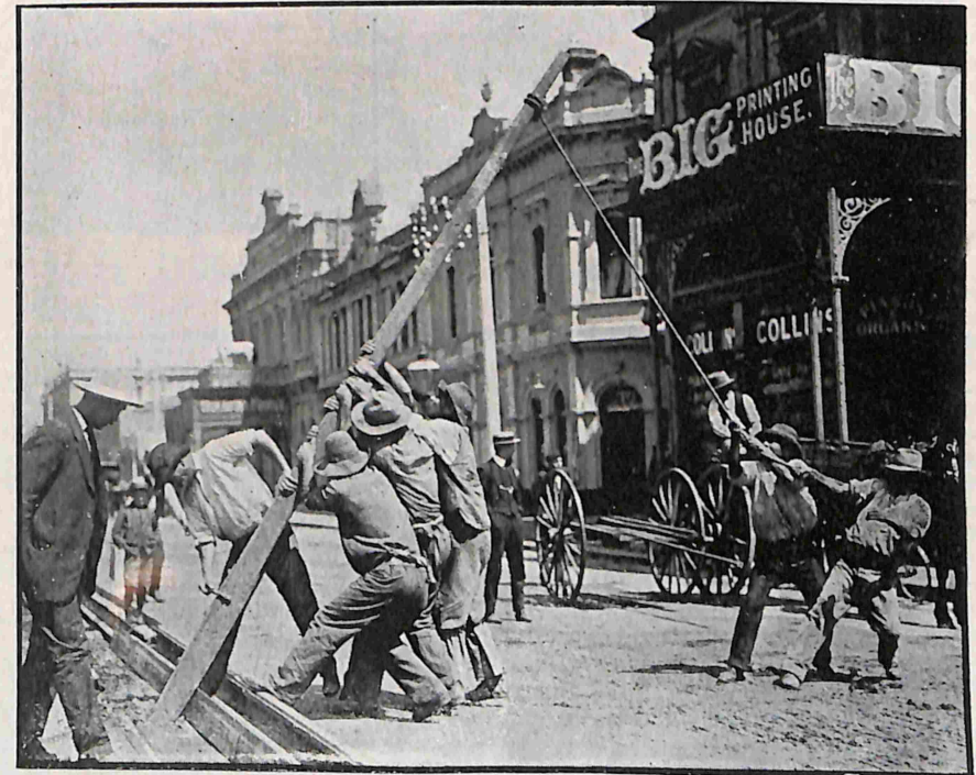
LIFTING THE OLD RAILS.
