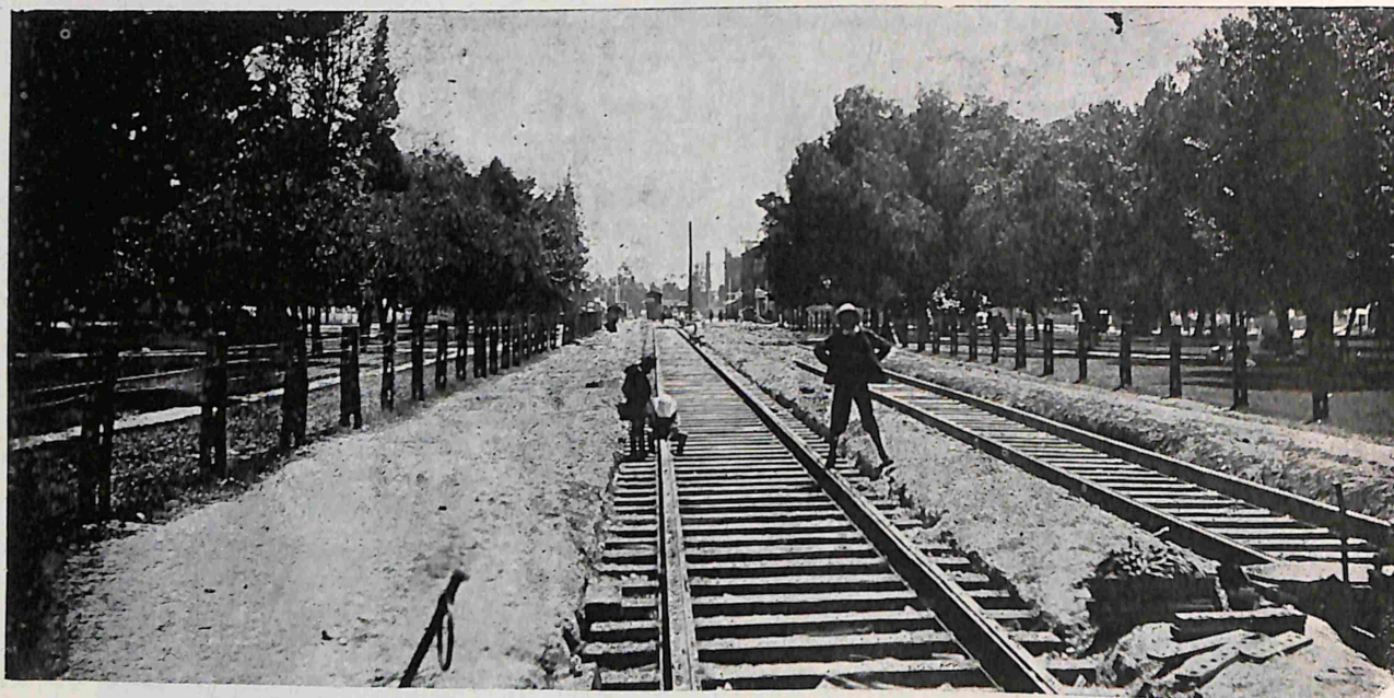
VIEW OF TRACKS FROM HINDMARSH SQUARE.
