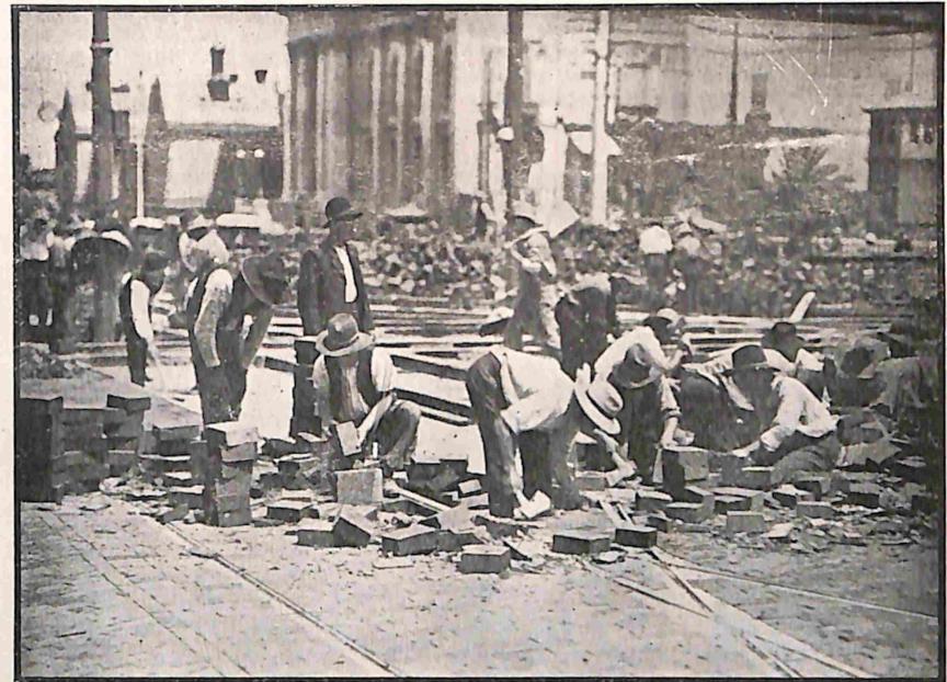
LAYING WOOD BLOCKS ON THE NEW TRAM TRACK AT THE BANK OF N.S.W. CORNER.
