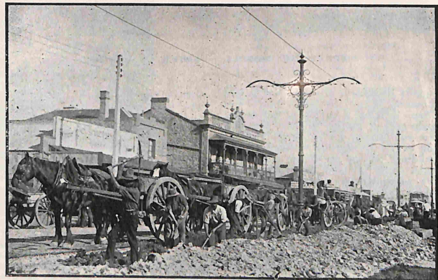
PUTTING IN THE NEW TRACK.
