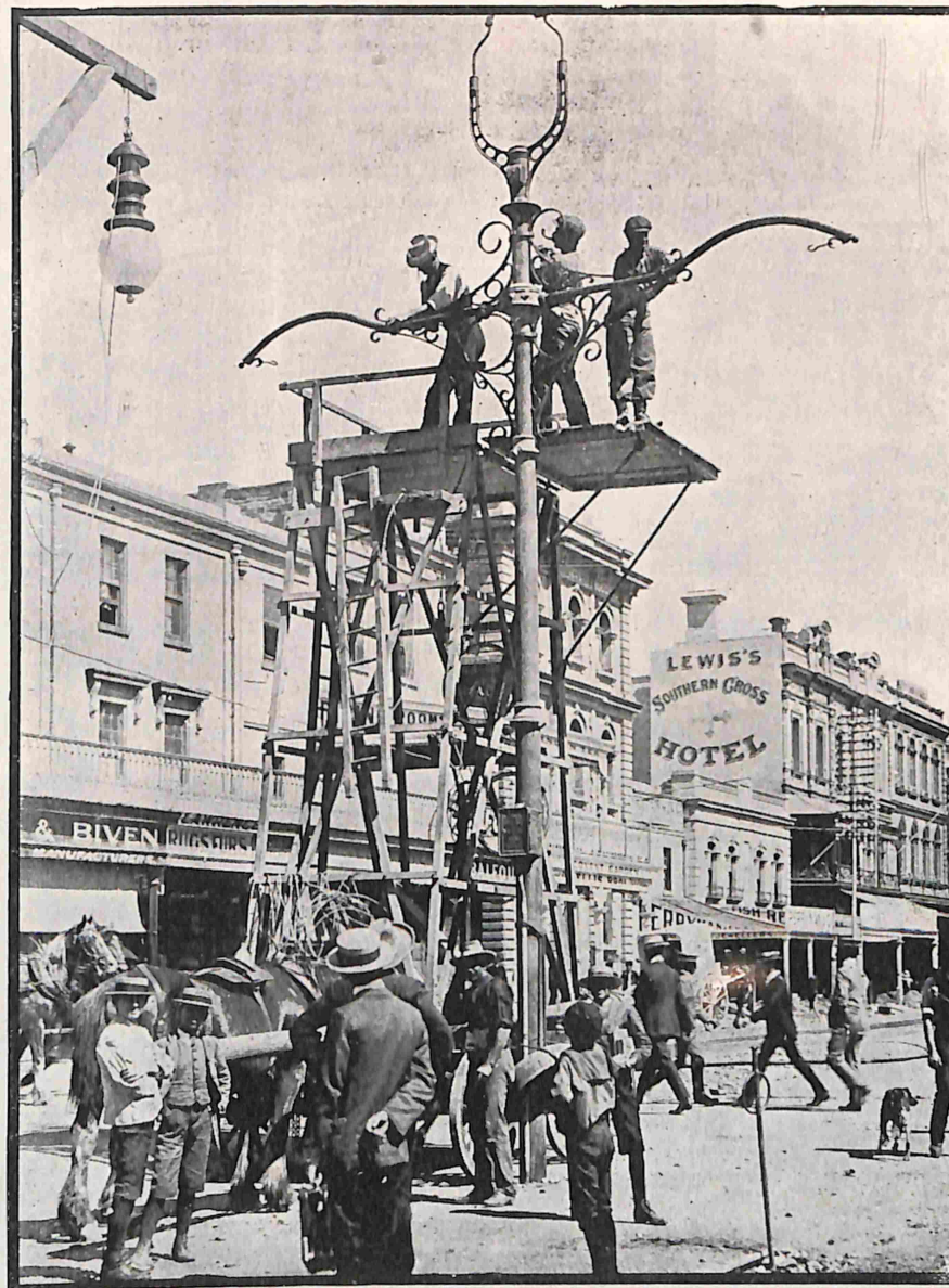
COMPLETING A COMBINED ELECTRIC LIGHT AND POWER CABLE POLE IN KING WILLIAM STREET.
