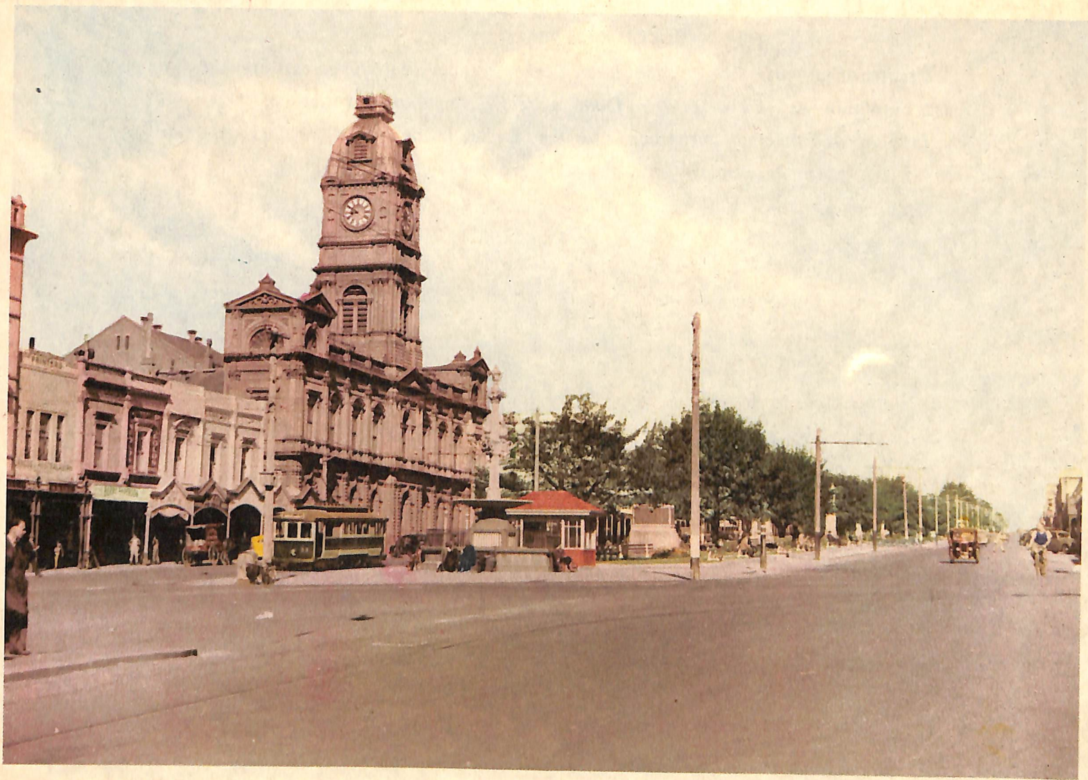
Another section of Sturt Street, one of the finest thoroughfares in Australia. This is only one of a number of streets in which are centered the business and commercial activities of the City.
