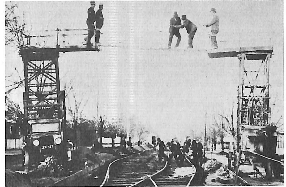
Replacing overhead and rails at Urquhart Street, Ballarat, in 1934. — S.E.C.
