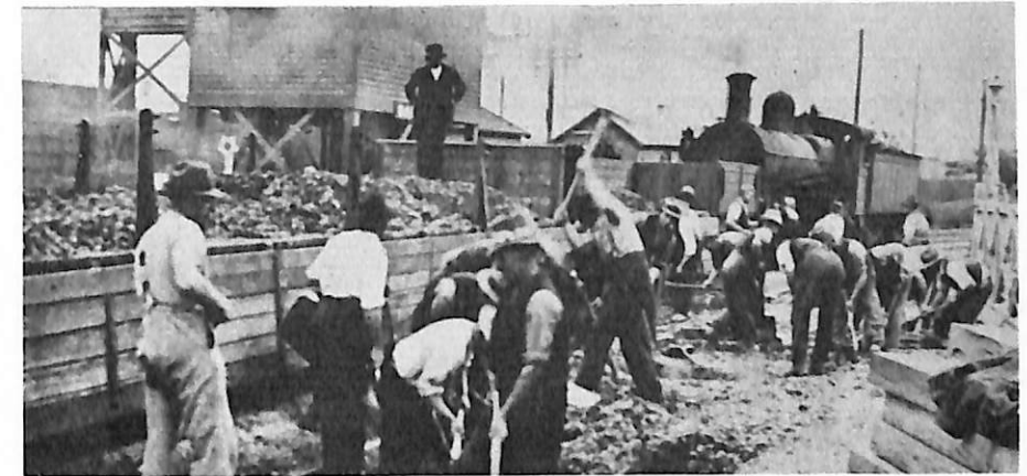
In 1934 the S.E.C. relayed the tramway / railway crossing in Lydiard Street North at Ballarat Station. The top photo shows the original crossing whilst the bottom photo shows workmen excavating this crossing. — Both photos S.E.C.
