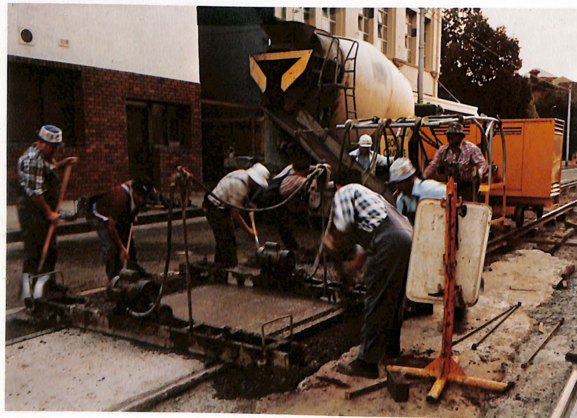
Civil Engineering team at work.
