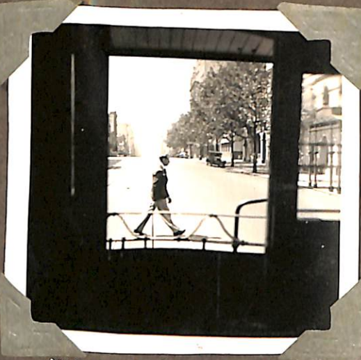
VIEW OF BOURKE ST FROM CABLE TRAILER.
