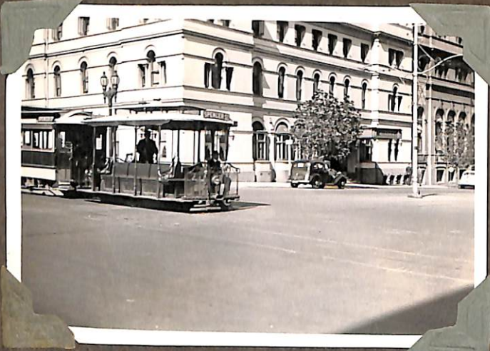
550 IN BOURKE ST. AT WILLIAM ST. MARCH, 1940.
