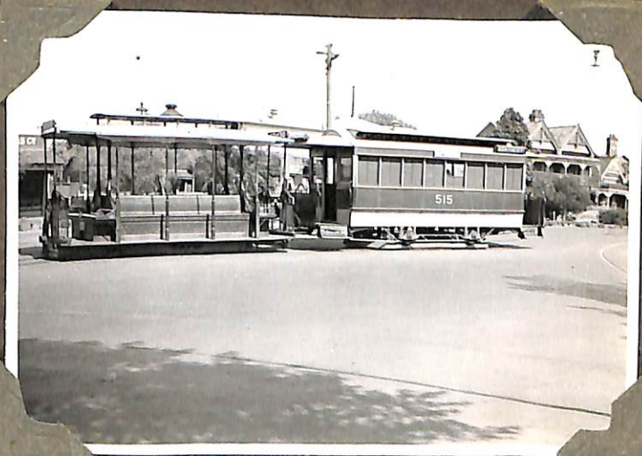
CABLE NO 515 OUTSIDE CLIFTON HILL TRAM DEPOT. 13-10-40.
