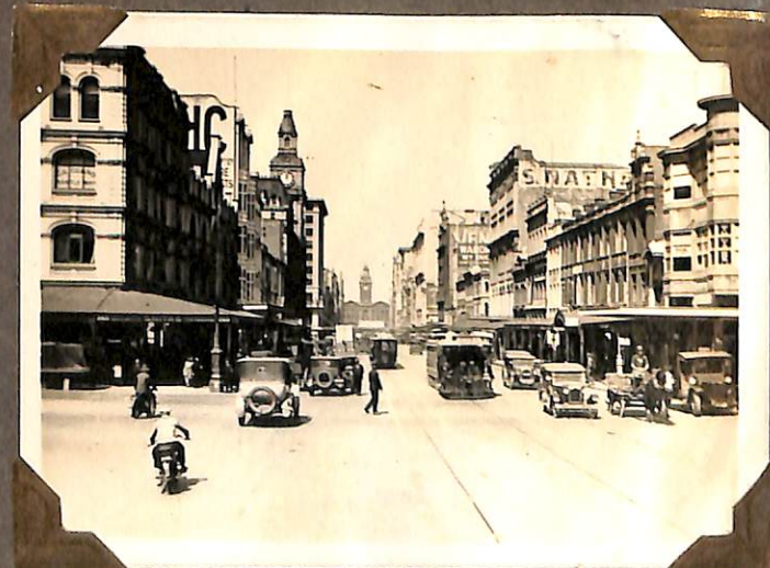
BRUNSWICK CABLES IN ELIZABETH ST.
