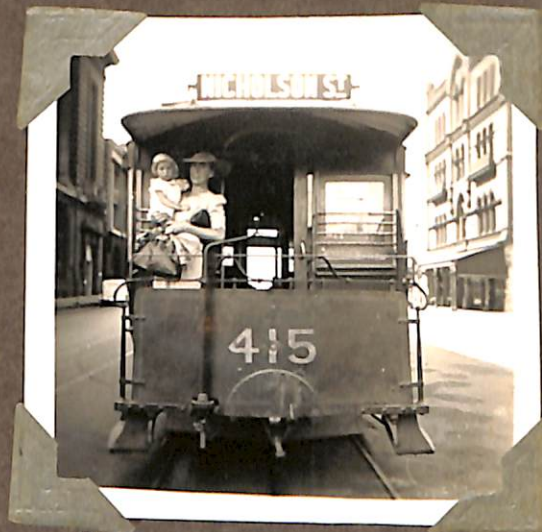
REAR VIEW OF CABLE BOURKE ST.
