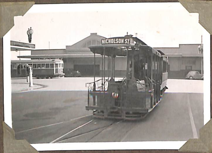
ELECTRIC & CABLE TRAMS. SPENCER & BOURKE STS.
