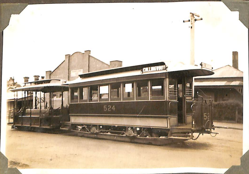
CABLE NO 524 AT COLLINGWOOD. TRAILER FITTED WITH SCRAPERS.
