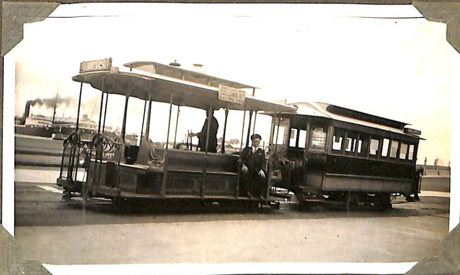
CABLE NO 449 AT PORT MELBOURNE TERMINUS.
