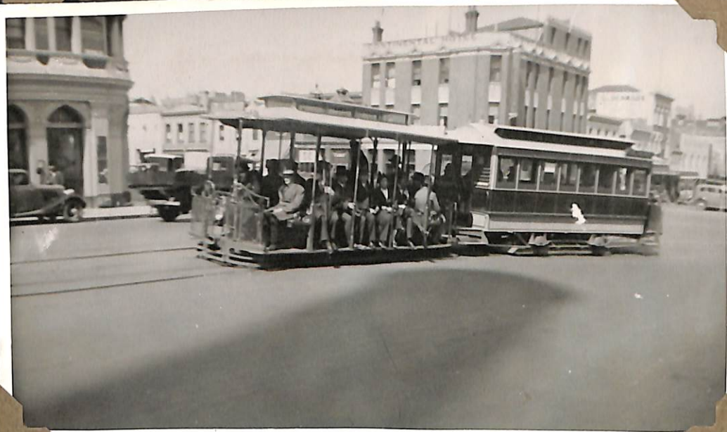
COLLINGWOOD CABLE NO 220 INTERSECTION OF RUSSELL & LONSDALE ST.
