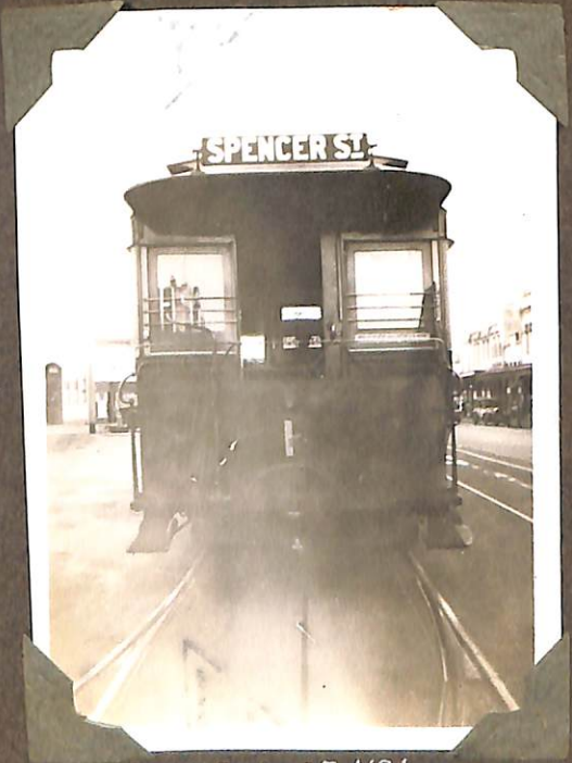
REAR VIEW OF NO. 1. NICHOLSON ST.
