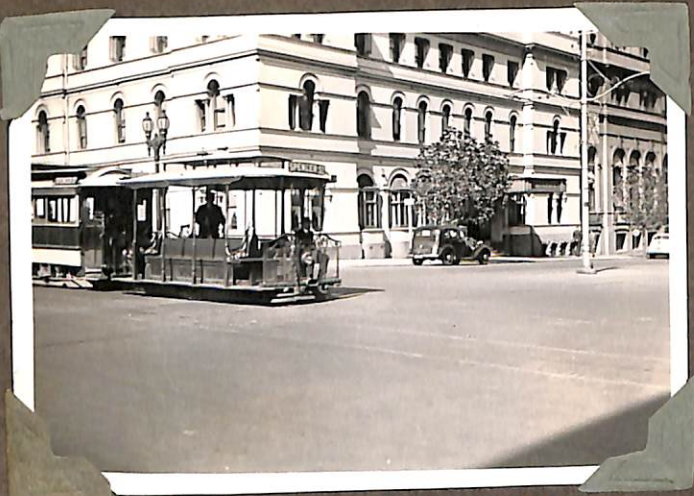
550 IN BOURKE ST. AT WILLIAM ST. MARCH, 1940.
