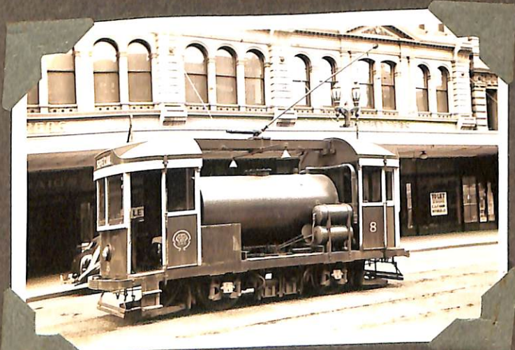
TANK CAR NO 8. BUILT 1934. ELIZABETH ST. CITY.
