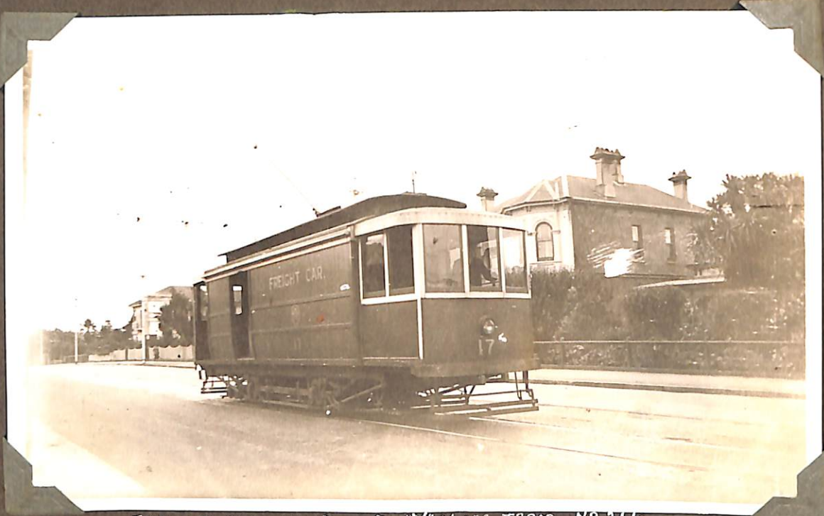
FREIGHT CAR NO 17. Ex "V" CLASS TRAM. NO 214 CONVERTED IN 1927. PHOTO TAKEN IN HAWTHORN.
