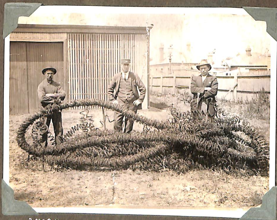
2700 FEET OF BUNCHED CABLE NTH. FITZROY DEPOT. 1918.
