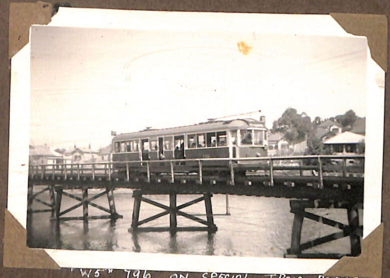
"W5" 996 ON SPECIAL TRAM BRIDGE OVER MARIBRYNONG RIVER.
