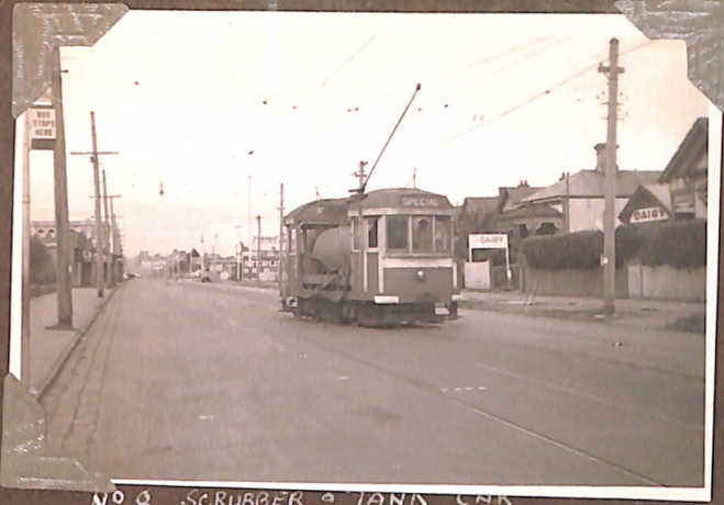
No 8 SCRUBBER & TANK CAR IN MARIBYRNONG ROAD 12-3-45
