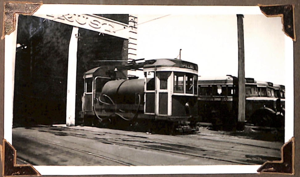
SCRUBBER NO. 8 AT FOOTSCRAY, JAN. 1950.
