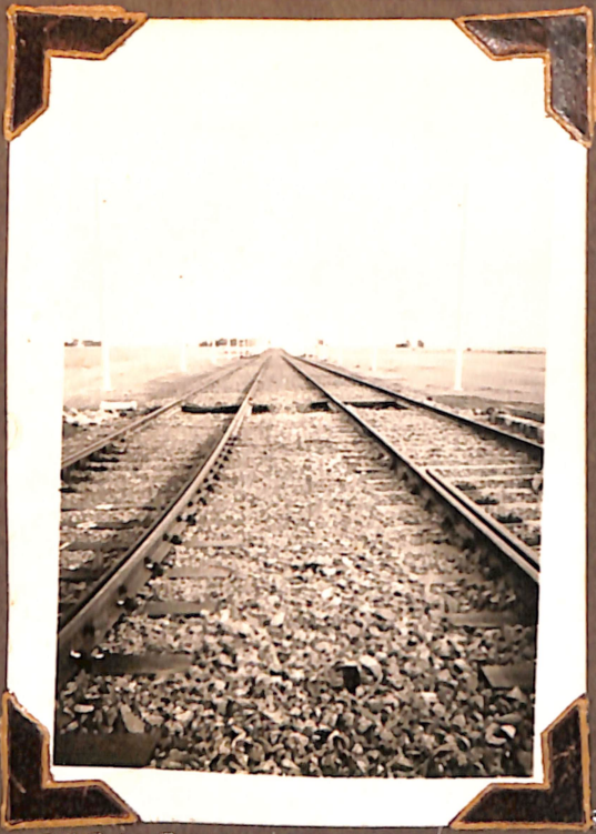
OPEN BALLAST TRACK TO ESSENDON DROME
