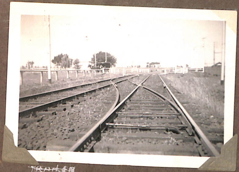
TRAILER TRAILING POINTS ON CROSSOVER ROYAL PARK.
