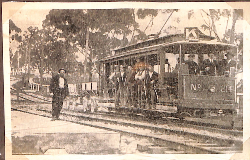
"V" CLASS NO 214 & BALLAST TRUCKS DURING BUILDING ON LINE THROUGH ROYAL PARK IN 1925. CAR NO 214 NOW NO 17 FREIGHT TRAM.
