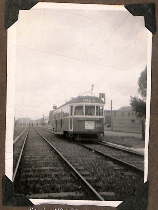
SW6 NO. 890 making trial trip over new Hanna St extension 21-12-44.
