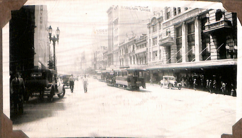
CABLES IN BOURKE ST. MELBOURNE.
