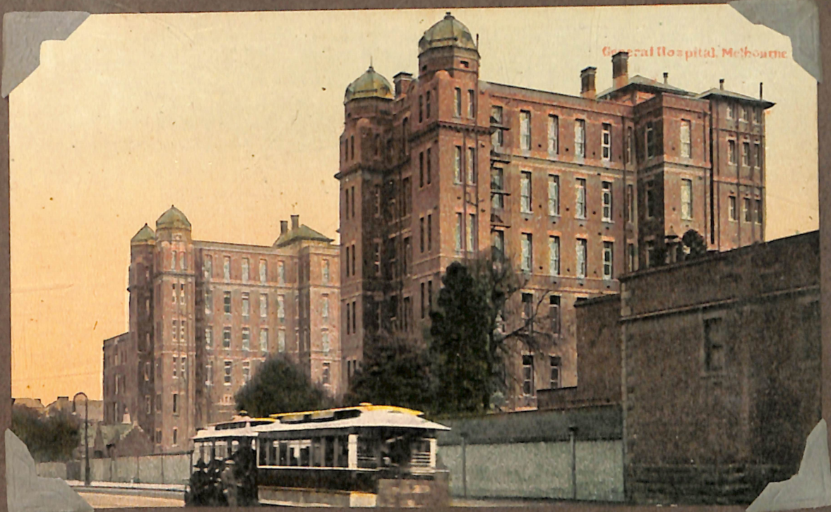
CABLE TRAM IN SWANSTON ST. LONSDALE STREET
