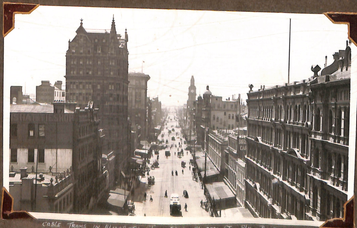
CABLE TRAMS IN ELIZABETH ST FROM FLINDERS ST RLY. BUILDINGS.
