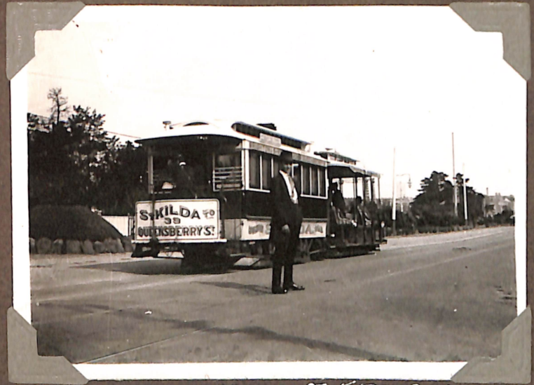
CABLE NO 39. IN ST KILDA ROAD NEAR ST KILDA JUNC.
