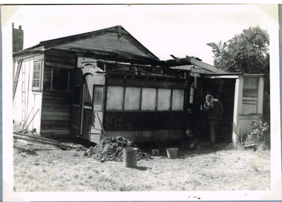
digging out N°3 Beaumain's horse farm 21/10/62
