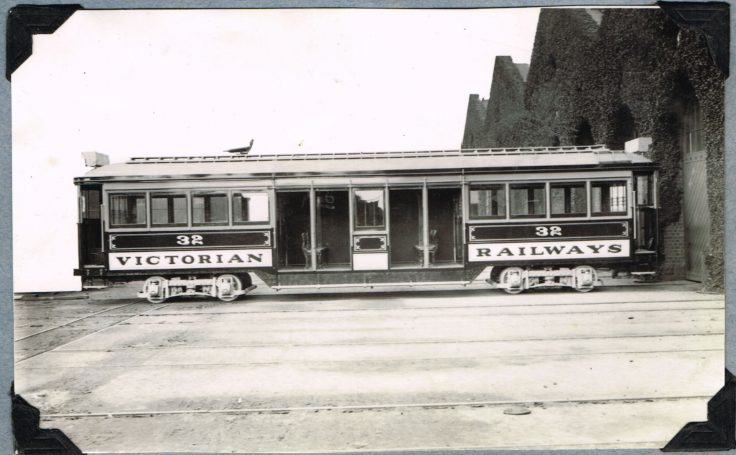
N°32 under construction NEWPORT RLY. SHOPS.
