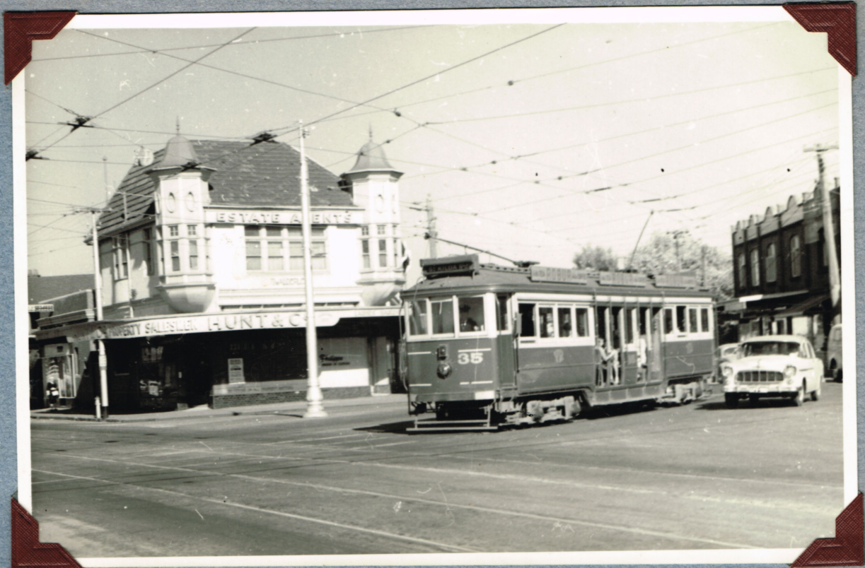
No. 35 INTERSECTION OF GLENAUNTLY & OSMOND RDS ELWOOD LAST DAY OF V.R. TRAMS 28-2-59.
