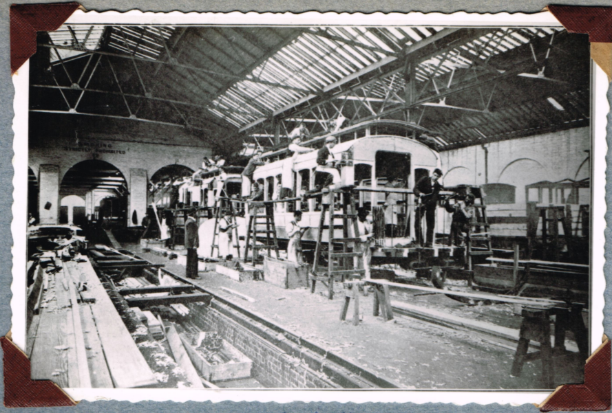
CONSTRUCTION of the first Nos 9 & 10 AT Newport Workshops about Aug 1906.
