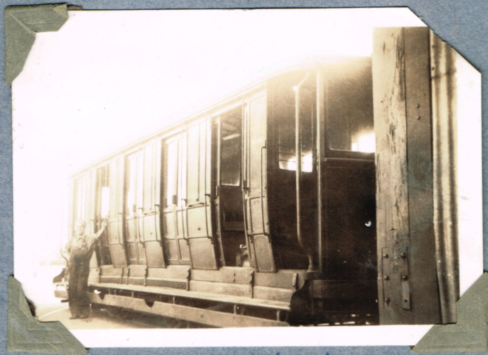
N o 20 as Works Tram Elwood depot.
