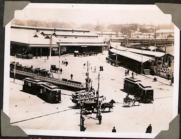
OLD SYDNEY RAILWAY STATION 1905 SHOWS D & C TYPE PERMANENTLY COUPLED SET. "D" 100 - "C" 17. ON LEFT. "C" 22 & 77 TRAILCAR ON RIGHT.
