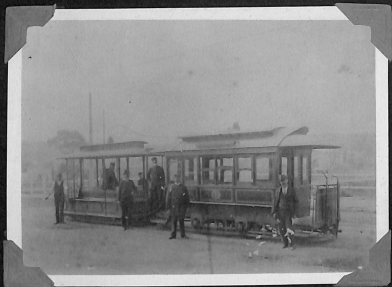
CABLE TRAM NO 17 RUSHCUTTERS BAY ABOUT 1904.
