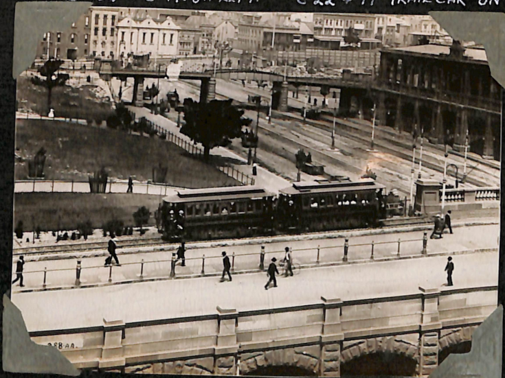
"C" TYPE NO. 87M AND 96T ON RLY. RAMP CROSSING OVER EDDY AVENUE.
