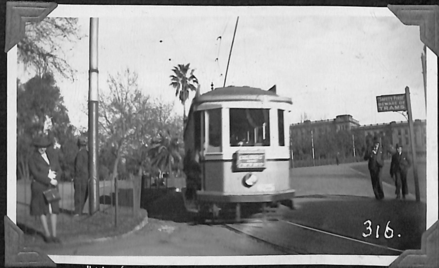
"N" 625 ON RAMP APPROACHING CENTRAL RAILWAY STATION SYDNEY
