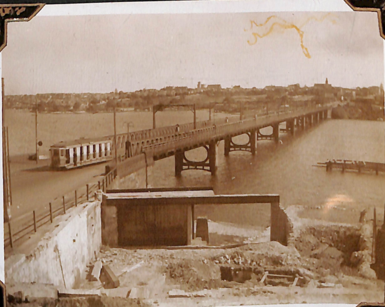
IRON COVE BRIDGE N CLASS 708.
