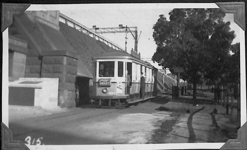
"N" CLASS 693 COMING DOWN RAMP FROM RAILWAY STATION.
