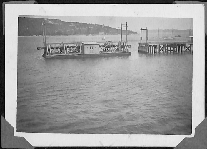
General view of tram punt Boxing Day 1938.
