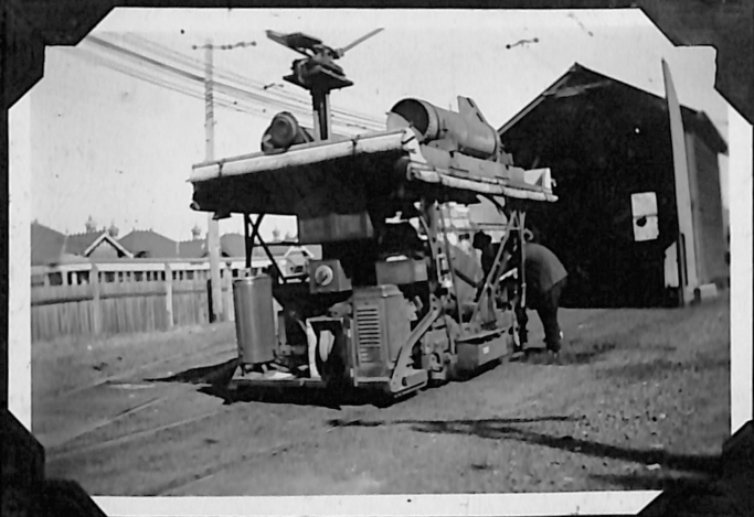
NO 3 RAIL GRINDER BEING FITTED WITH NEW BELTS. DEC. 1937.
