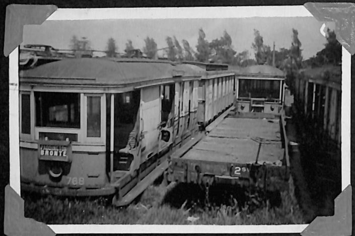
K 768 WITH EYE TESTING CAR N°125 BEHIND BALLAST TRAILER 29 RANDWICK SHOPS
