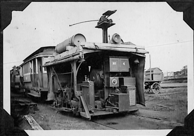
NO 4 RAIL GRINDER AT ST. LEONARDS RAILWAY GOODS YARDS & TRAMWAY PERMANENTWAY DEPOT JULY 1939.
