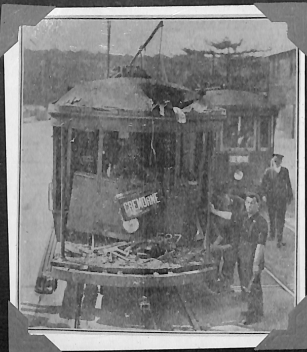
"E" CLASS 527 SHOWS DAMAGED CABIN THE SPIT. 7-12-1933
