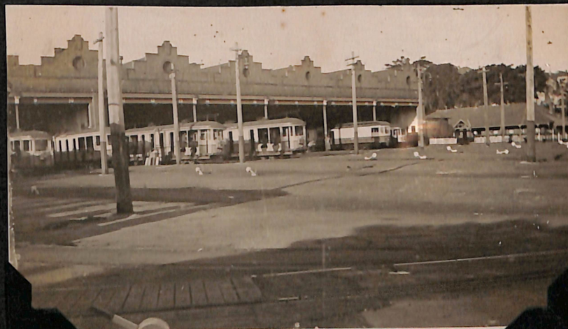
"O" class 41 service car Rozelle depot. held safely 160 cars on 25 roads.
