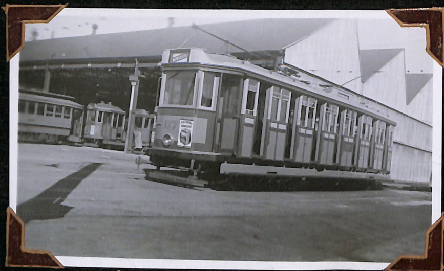
LP N o 177 GORDON AVE DEPOT 28-8-47 CAR OUT FROM PAINT SHOP.
