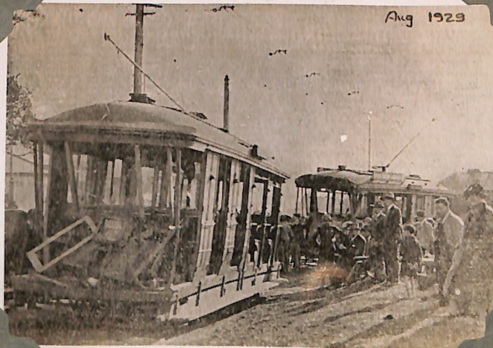
Aug 1929 Result of smash on single line between Park and Gap loops Watson's Bay line Aug. 1929. "K" CLASS TRAMS.
