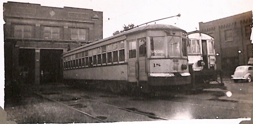
STARK ELECTRIC No. 18 CANTON, OHIO.
