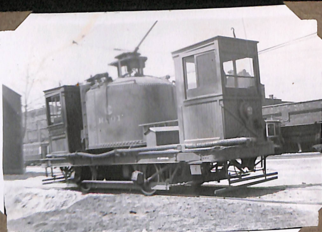
CHICAGO SURFACE LINES. No. R201 SAND CAR AT WENTWORTH DEPOT.
