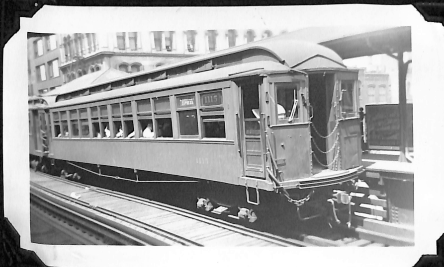
CHICAGO RAPID TRANSIT TRAILER ON ELEVATED RAILWAY.
