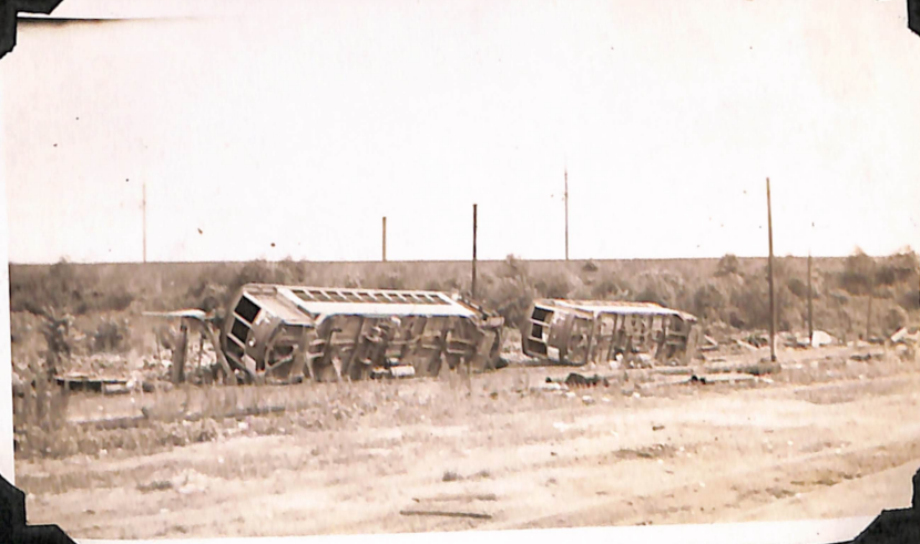
SCRAPPING CARS ON NEW YORK & QUEENS LINE
