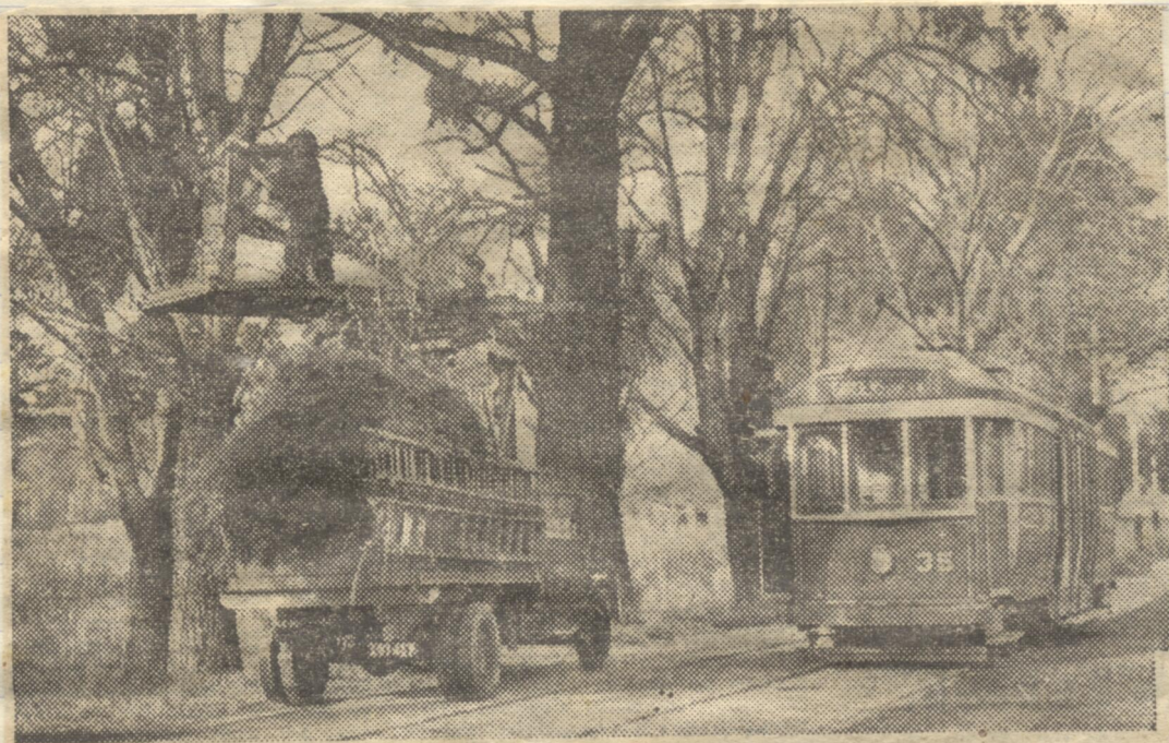
Ballarat trees add beauty to the city but they must be kept in their place. Pictured above are SEC men lopping branches that threaten to interfere with overhead wires of the tram track in the vicinity of Lake Wendouree.
