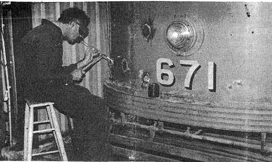
Warren Doubleday welds up the old advertising holes on No. 2 end of 671; 5.1.92. Photo Len Millar
