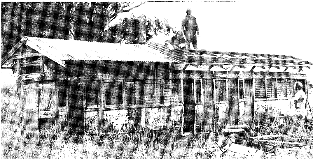
Removing the roof from No. 121 at Bungaree, Oct 29, 1994. PHOTO: Carolyn Dean.
