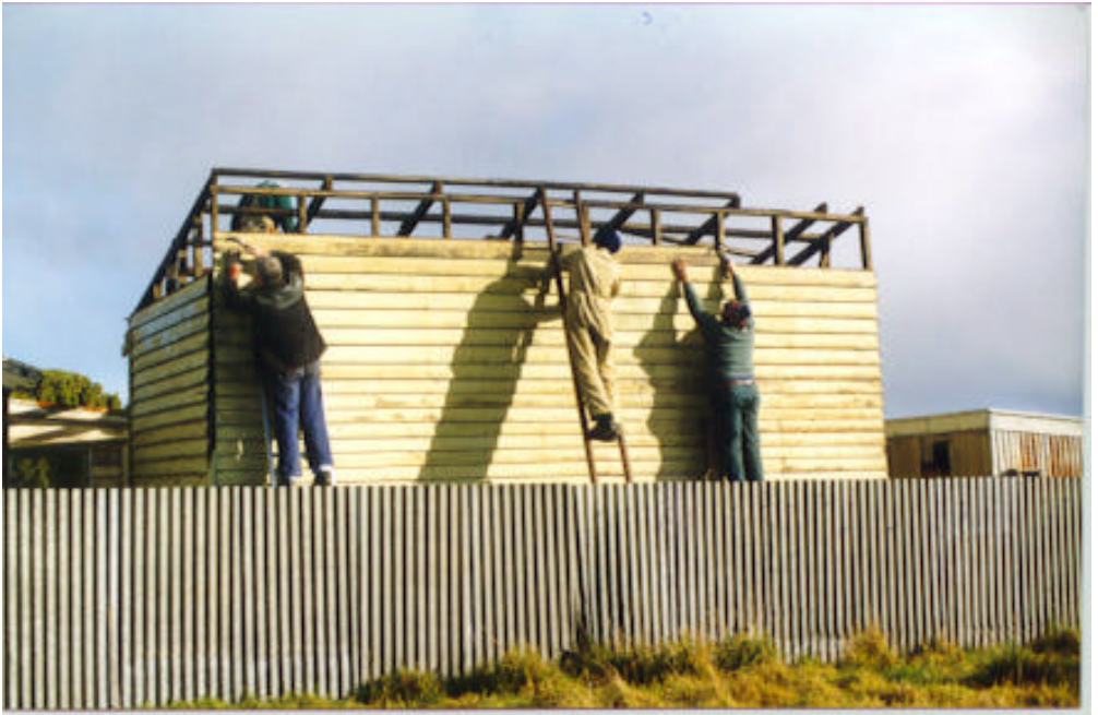
Putting the weather boards back on during a Sunny break on 15 May 1999. In the photo are Peter Winspur, Simon Jenkins and Alan Snowball. John Phillips is on the roof. Photo Carolyn Dean.
