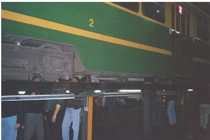
Inspecting the underside of Z2 at Southbank depot on Sat. June 5. Er's where the compressor?
