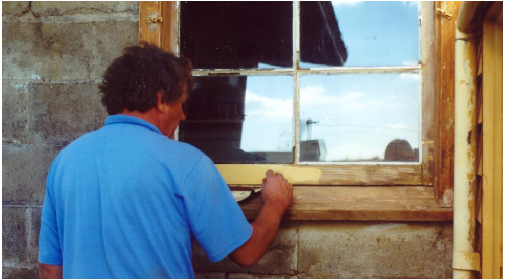
Jim Parker puts the first coat on to one of the house windows after rubbing it down and removing all the old paint - 8 April 2000. Photo Carolyn Dean
