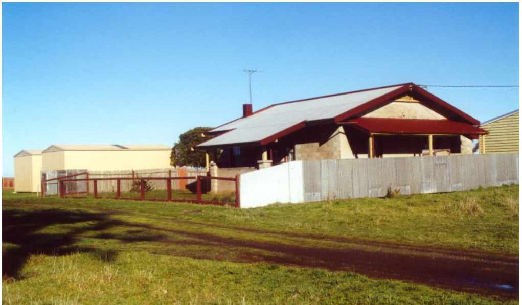
Bungaree house looking much more presentable in its new paint and with the two completed sheds behind. Photo Carolyn Dean 11/6/2000.
