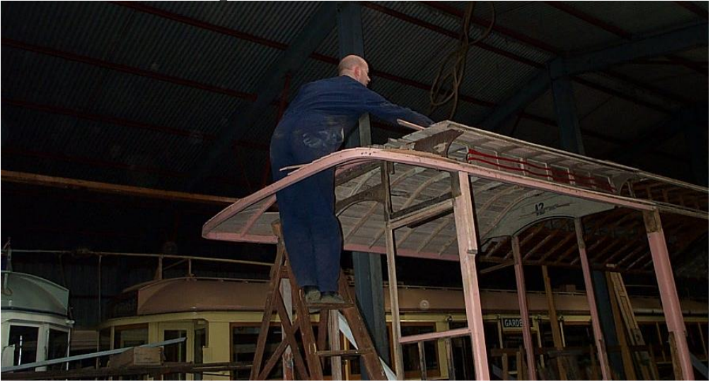
Gary Wood fits another sanded and primed roof slat to No. 12.
