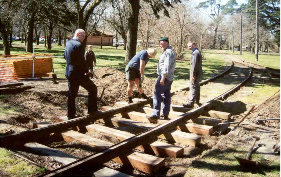
Our track gang replacing sleepers at the depot level crossing on the lead to number 2 and 3 roads. Garry Wood, Daniel Edwards, Alan Snowball and Greg Histen are hard at it while the President poses for the camera. Saturday 14/9/02. Photo: Warren Doubleday
