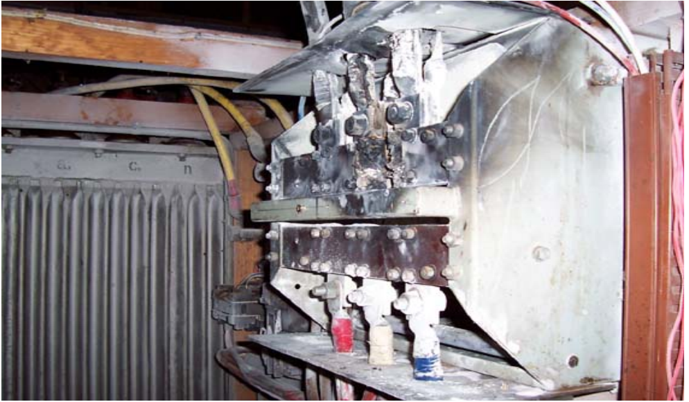
Above: The old main traction power switch – after the fire. 19 October 2004. PAUL MONG
